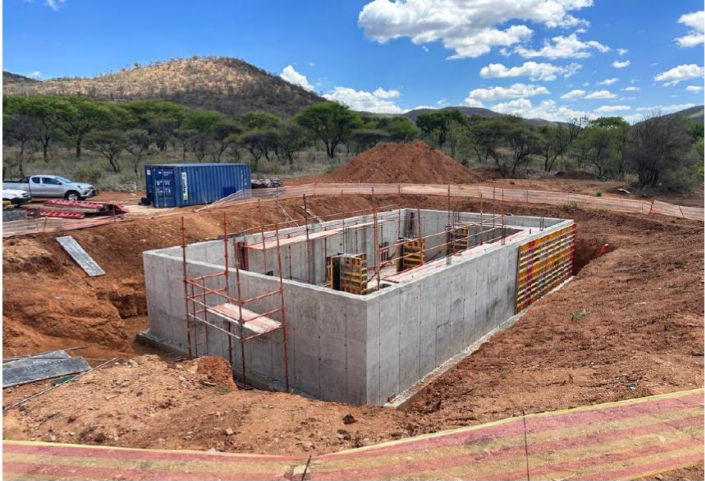
Pump Station 1 Concrete to Walls & Columns
