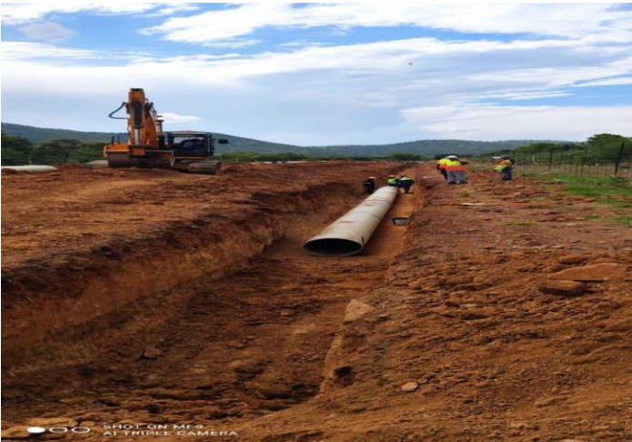
Laying of pipeline from Loskop to Pump station 1 Source: Department of water and sanitation
